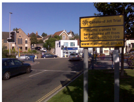
Cabstand junction before signal switch-off
