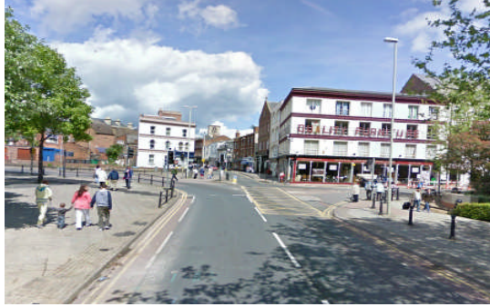
Kimbrose Way, Gloucester – before
